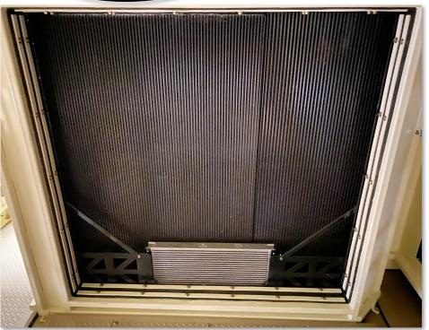
The Caterpillar bar and plate cooler has slightly more square inches of jacket water core face area than the Copper Core equivalent.
